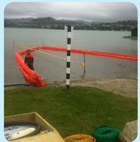
Getting ready to put the boom for constraining oil spills into the inlet
