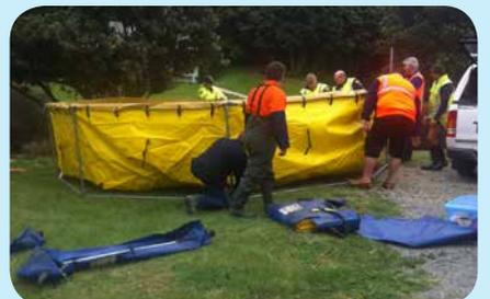
Holding pool for oil in a potential spill
