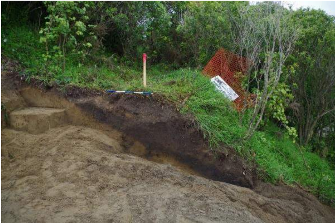
Figure 38: Upper track in eastern edge of alignment, shows deposit of fill to form track bench, 1 metre scale (17 September 2015).
