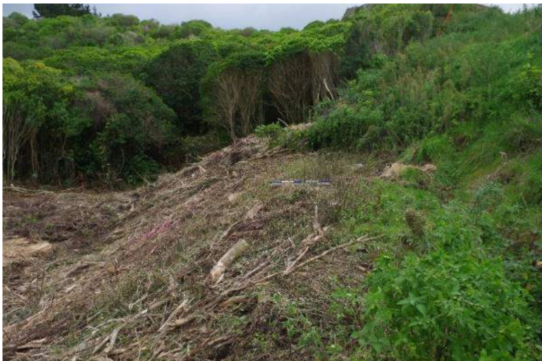
Figure 37: Lower track exposed on western edge of expressway alignment, 1 metre scale (12 June 2015).
