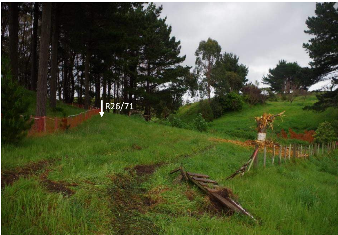
Figure 87: Looking south towards site prior to excavation for road cutting (07 October 2016)
