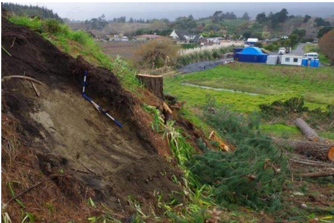
Figure 47: Re-deposited midden (not sampled) between track cuttings 1.0 + 0.5 metre scale (1 August 2014).
