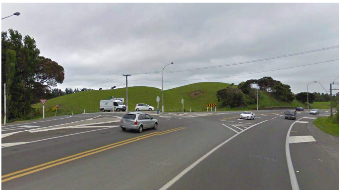
Figure 98: Dune as seen from SH1, looking north, prior to earthworks
